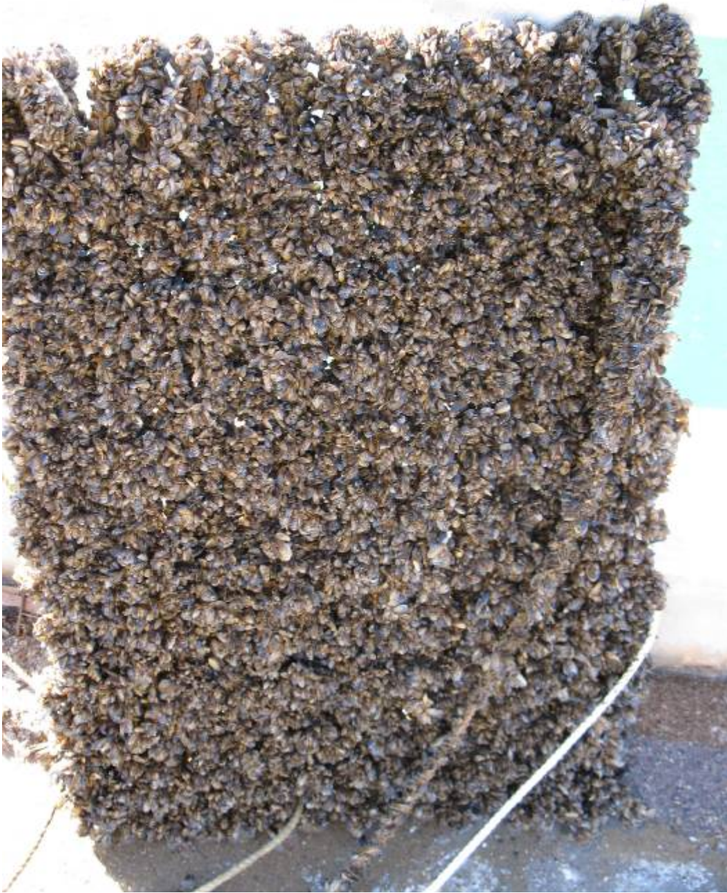
Figure 4.—Uncoated steel after 7 months of exposure in dynamic conditions. Test period May 2008 to December 2008.
