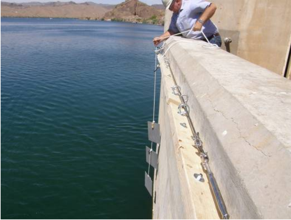
Figure 2.—Coated steel plates placed in static exposure from the face of Parker Dam.
