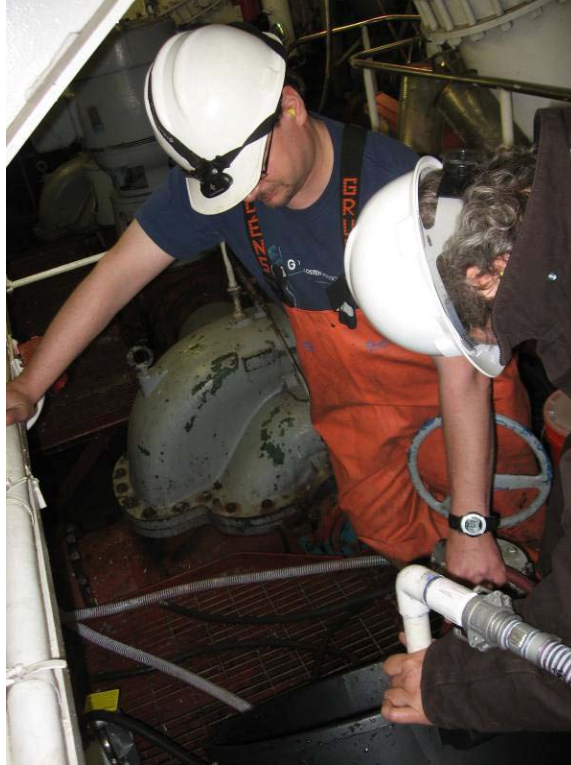
Photo 9 Making Discharge Sampling Connection
