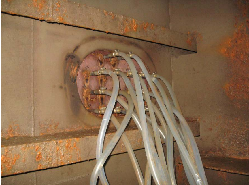
Photo 6 Discrete Tubing Internal Terminations—Steel plate located in ballast tank bulkhead where all discrete tubes for that tank are terminated (view from inside ballast tank)
